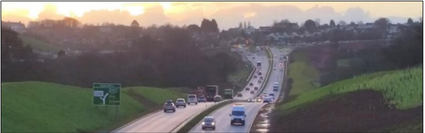
Figure 17 South Devon Highway completed scheme
